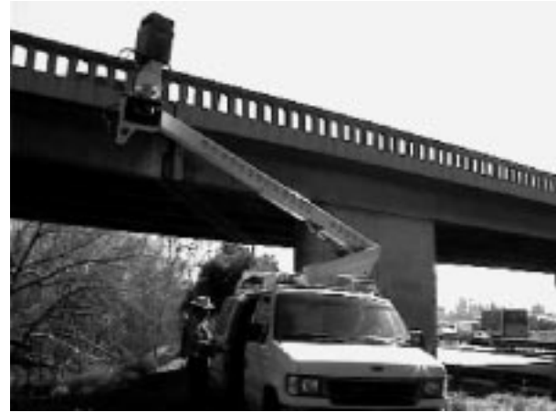
Highway Widening Project Using Laser Scanning (Mark Thomas & Co. project)
