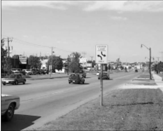
South Duff Avenue in Ames, Iowa, after retrofit in 1994 with a continuous TWLTL (five lanes) and a driveway management and consolidation program. After completion of the project, the crash rate fell by about 70 percent and traffic operations improved one full level of service even though traffic volumes increased seven percent.
