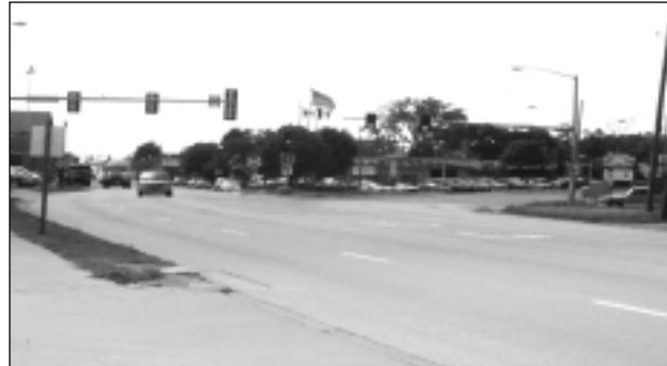
State Street (US 67) in Bettendorf, Iowa, after retrofit in 1996 with a continuous TWLTL (five lanes). After completion of the project, the crash rate fell by more than one-half and traffic operations improved one full level of service even though traffic volumes increased eight percent.
