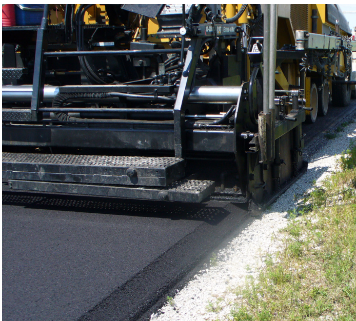
Hot-mix asphalt application of the Safety Edge on rural roadway
