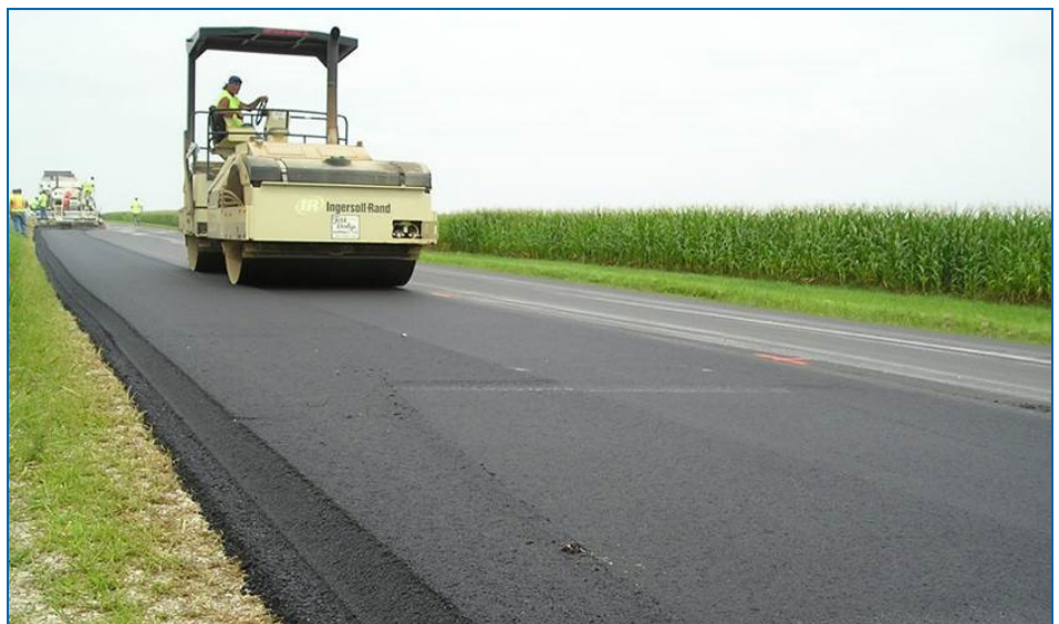
Placement of Safety Edge by asphalt paving operation
