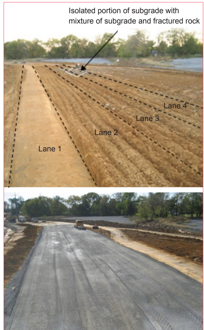
Figure 3. Subgrade test strip layout (top) and base layer (bottom)
