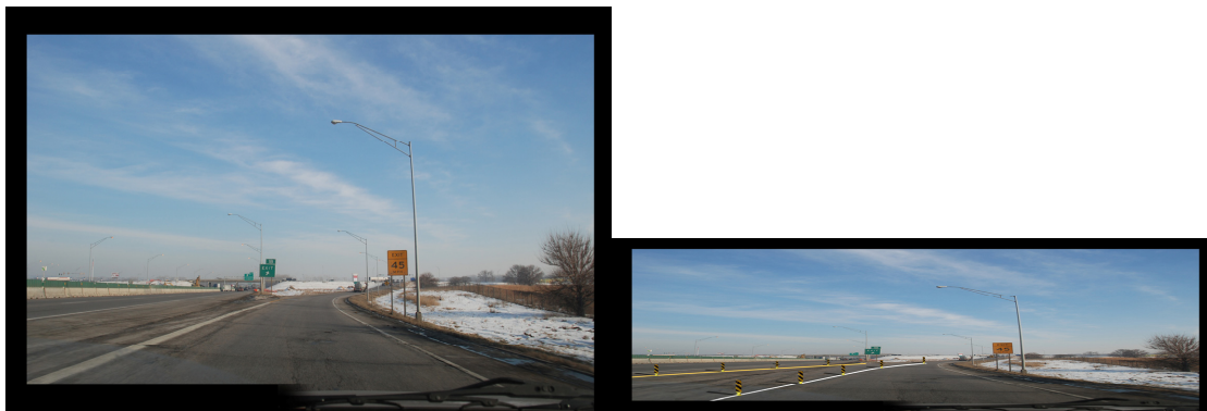
Figure 2. Original ramp (left) and traffic image retouched (right) on southwest ramp merging onto 24th Street
