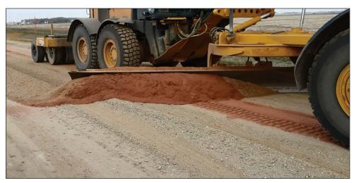
Researchers used motor graders to blend crusher dust with loose aggregate floating on the road surface. This was intended to restore fines that bind the aggregate. The effectiveness of the procedure depended on the plasticity of the available crusher dust.
