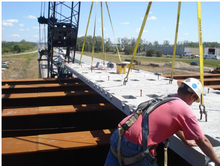
**Figure 2.5. Placing precast deck panel on girders**
