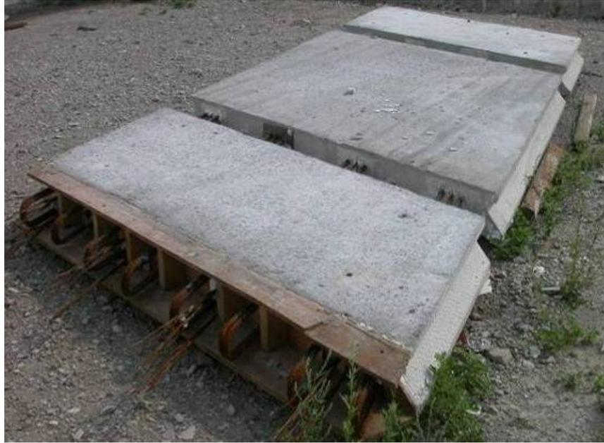
**Figure 1.1. Boone County precast concrete deck panel (Wipf, et al. 2009)**
