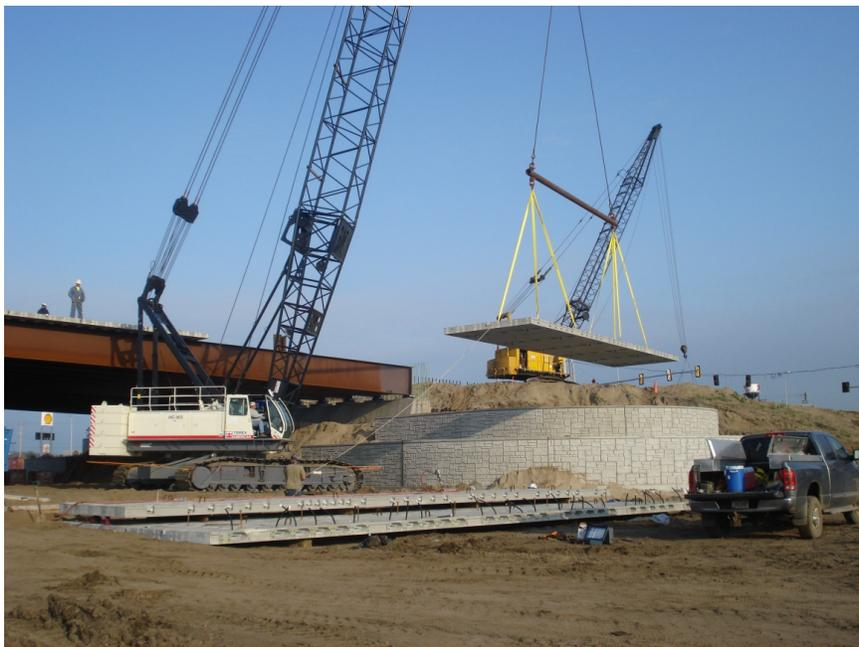
**Figure 4.5. Deck panel being lifted into place**
