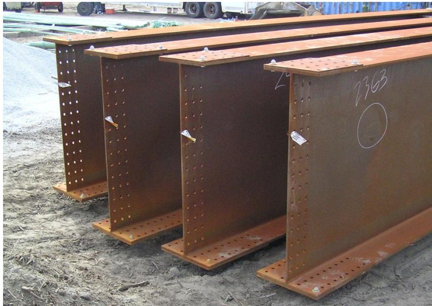
**Figure 2.3. Girder ends at field splice location**
