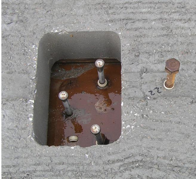
**Figure 2.8. Shear stud pocket and studs**
