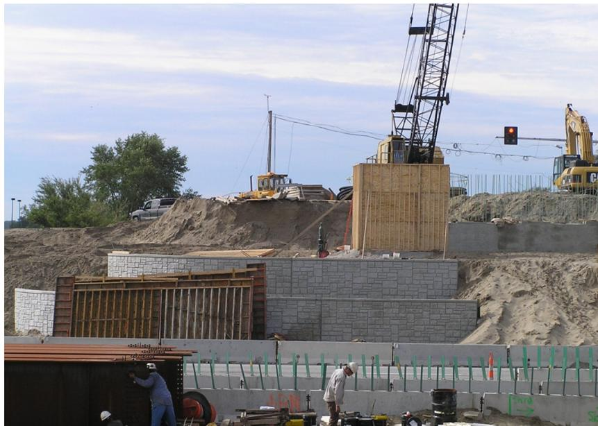
**Figure 2.1. Construction of south abutment and terrace walls**
