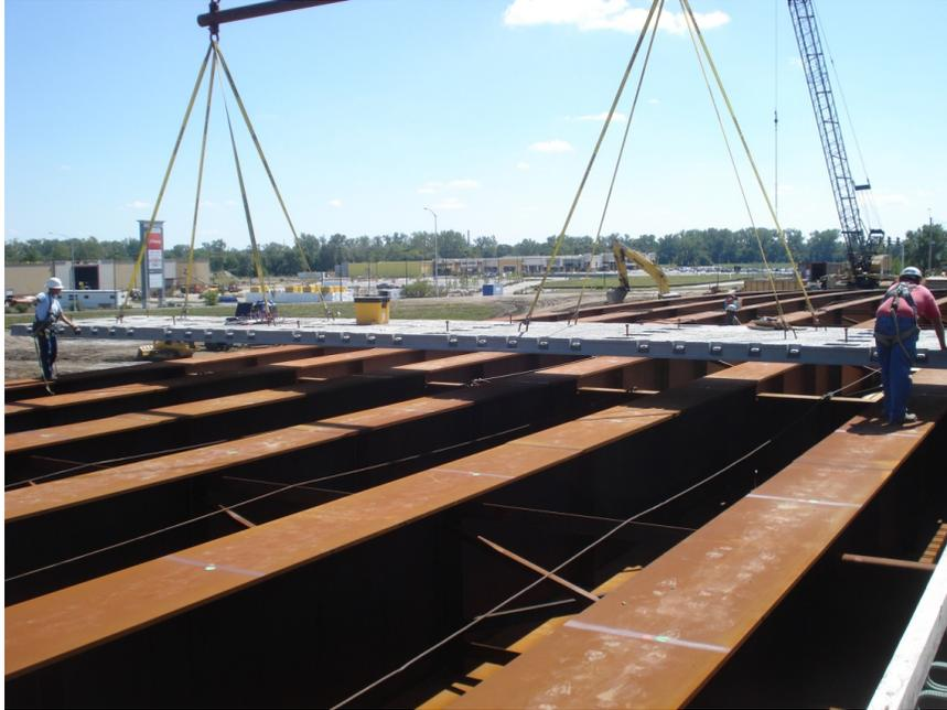
**Figure 4.6. Final maneuvering of precast deck panel placement**
