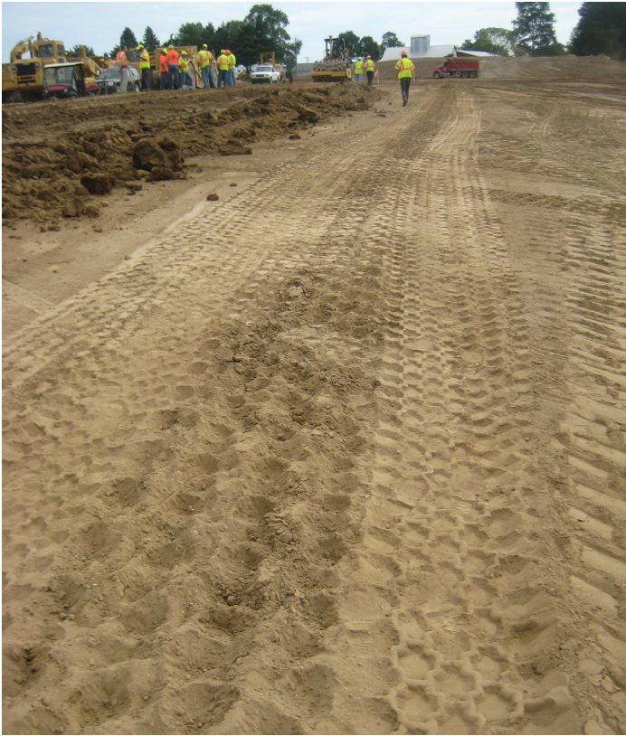
Figure 2. TB5 cohesive embankment fill test strip (from White et al. 2011)
