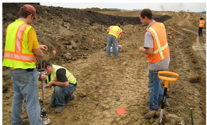
Figure 3. Test strip 2 construction and testing (from White et al. 2009)
