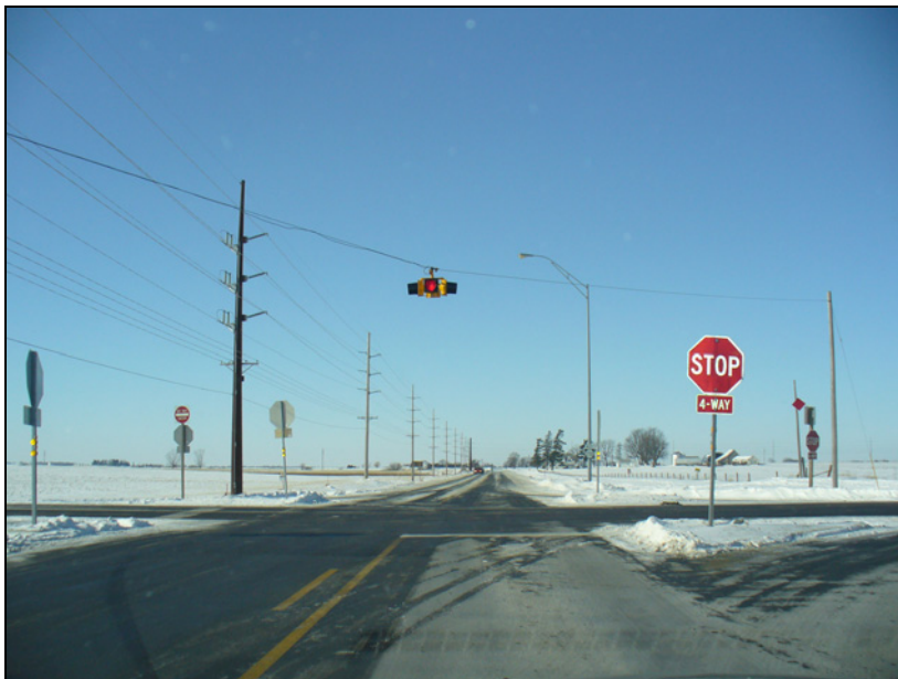
Figure 9. Use of overhead flashing beacons at all-way stop intersections (Image source: Neal Hawkins)
