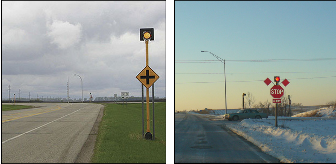
Figure 4. The Minnesota DOT's sign-mounted beacons used to replace overhead flashing beacons (Right image source: Mn/DOT from Amparano and Morena, 2006, Left image source: CTRE)
