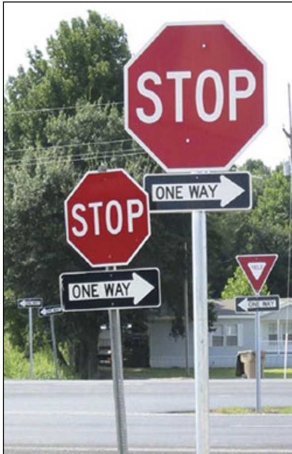
Figure 7. Mississippi DOT upgrades of sign size (Image source: MDOT from Amparano and Morena 2006)
