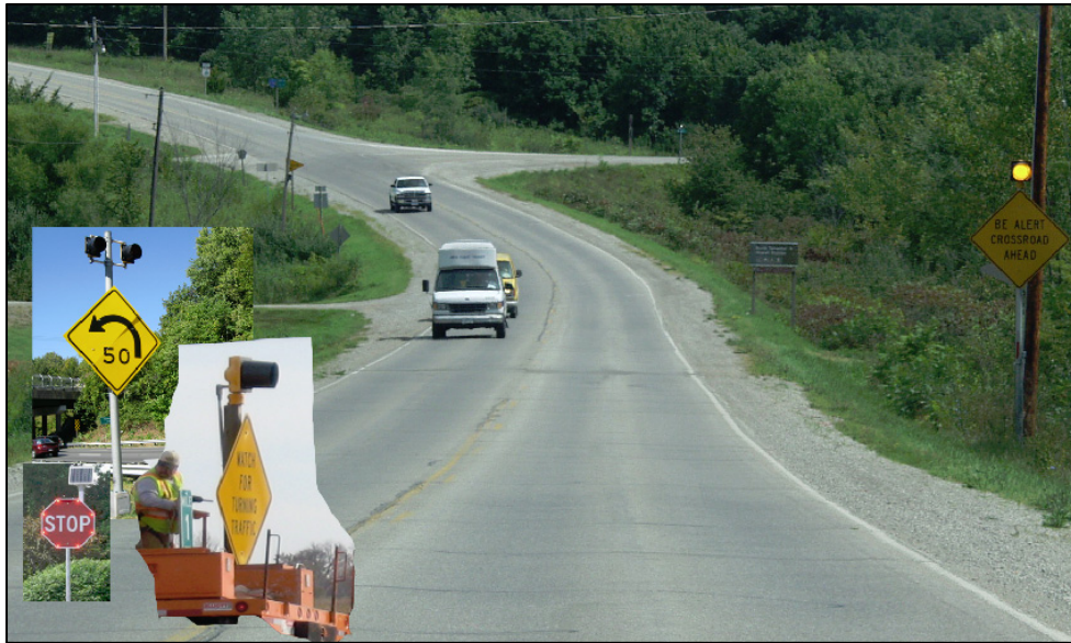
Figure 3. Flashing beacons in a variety of settings (Image source for LED Stop Sign: TAPCO, all other images Neal Hawkins)
