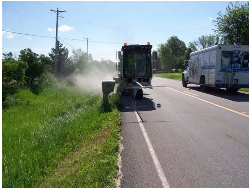
Figure 3-13. Milling operation omitting short areas around mailboxes in Polk County
