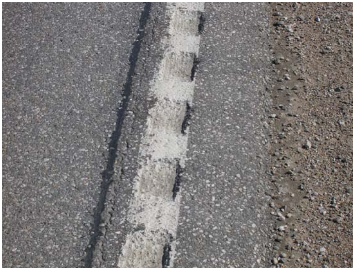
Figure 5-15. Similar wear for rumble stripe and flat section (taken spring 2009). F-29 is on the left and P-53 is on the right.
