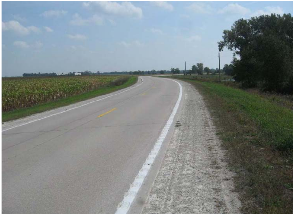
Figure 4-3. Rumble stripe installation on W-13 (photo courtesy of Neal Hawkins, CTRE)
