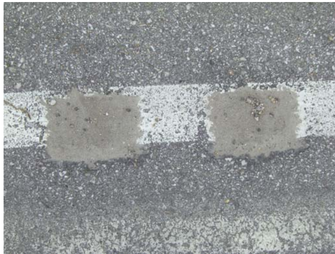
Figure 5-3. Rumble stripe with caked fines in bottom
