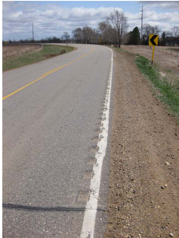
Figure 4-15. Rumble stripes on B-30
