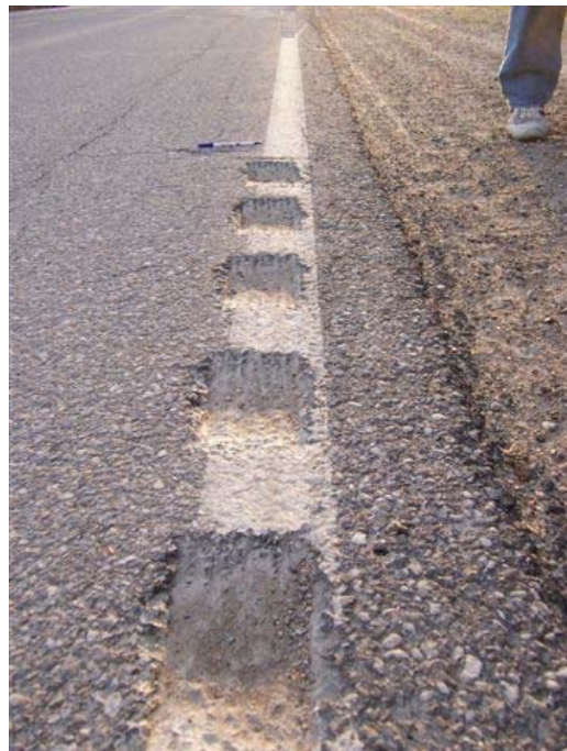
Figure 5-17. Another portion of F-29 showing less wear in the rumble stripe than in the flat area (taken spring 2009)
