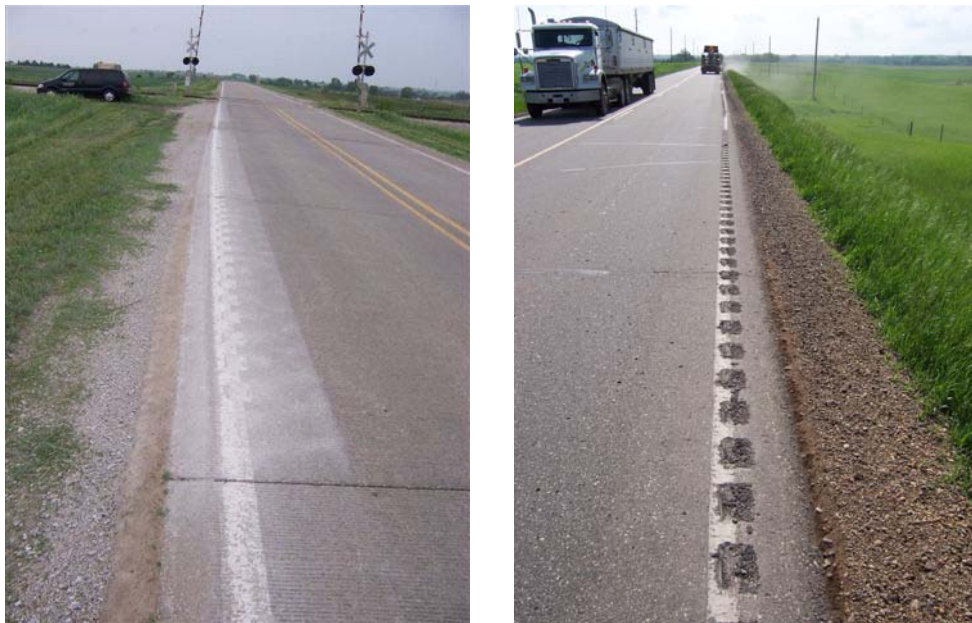
Figure 3-9. Examples of milling work
