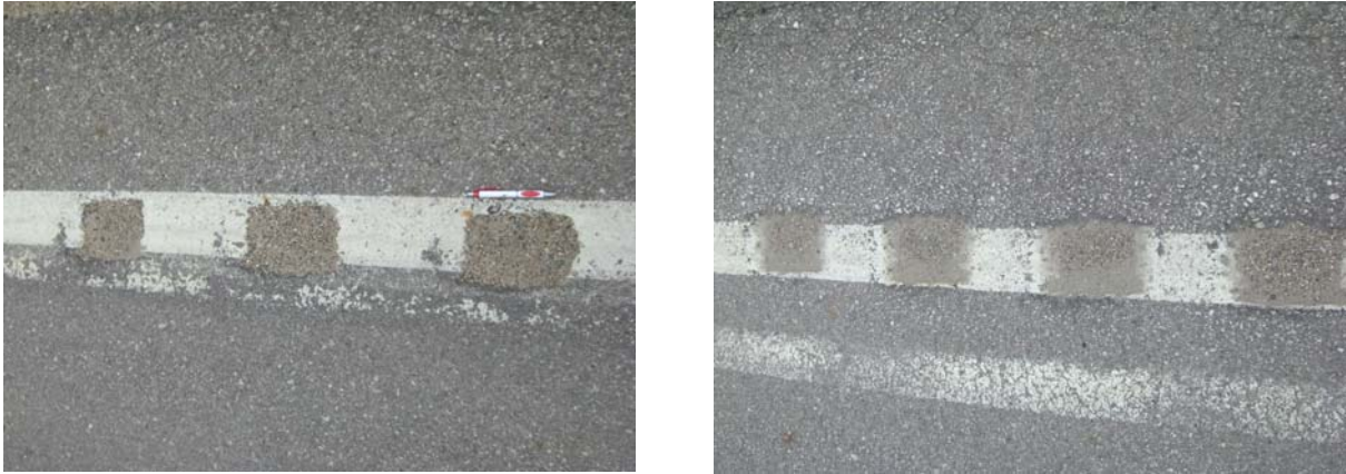
Figure 5-2. Rumble stripes filled with sand
