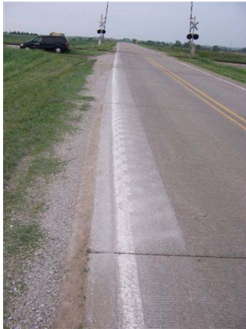
Figure 4-6. Rumble stripe installation on P-53
