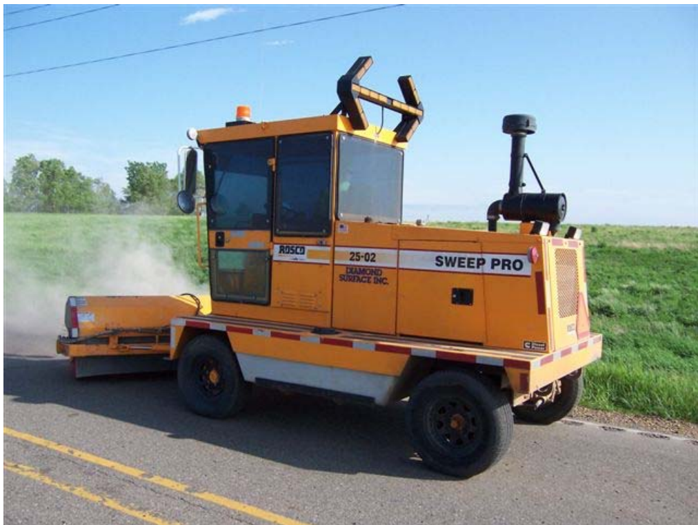
Figure 3-6. Machine sweeping completed rumble strips after milling
