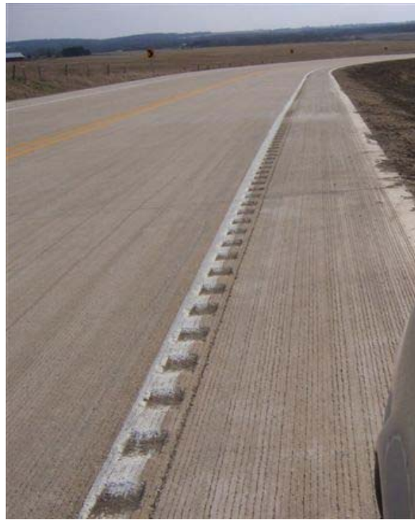
Figure 4-18. Rumble stripe installation on E-16
