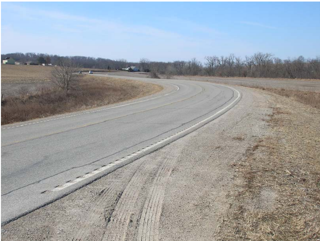
Figure 4-12. Rumble stripe installation on F-29
