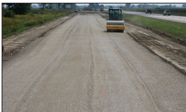
Figure 5. Mapping operations on a production base layer test production test bed (from White et al. 2010)
