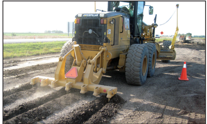
Figure 3. Preparation of calibration test beds (from White et al. 2010)
