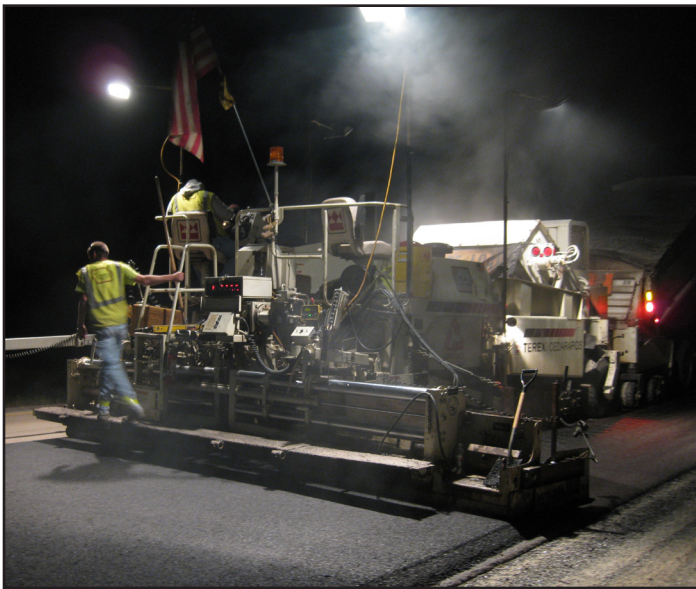
Figure 1. Paving operations on US218 project (from White et al. 2010)
