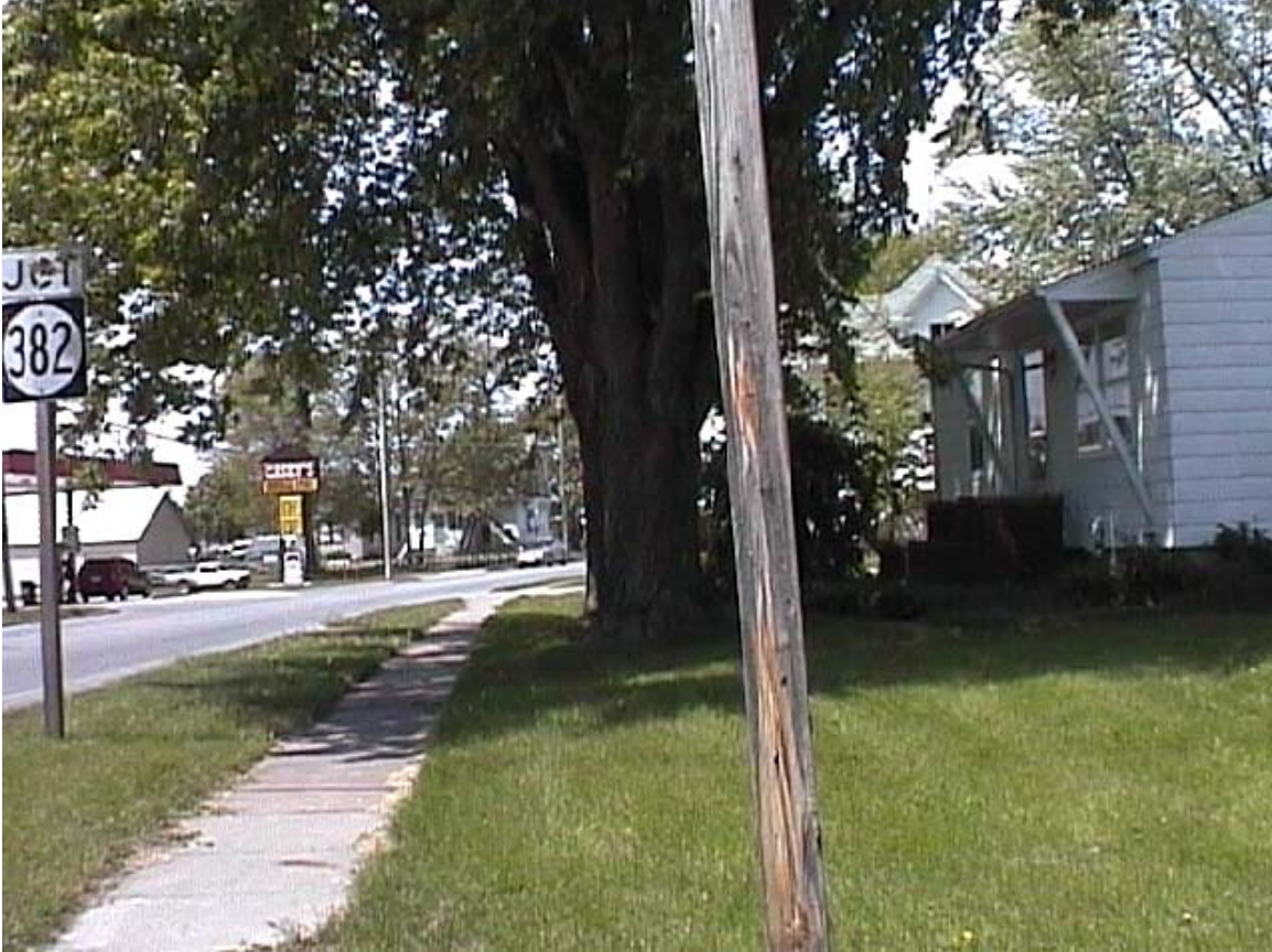
Figure C.2. Stopped driver's view at the intersection of Market St. and E. First St.
