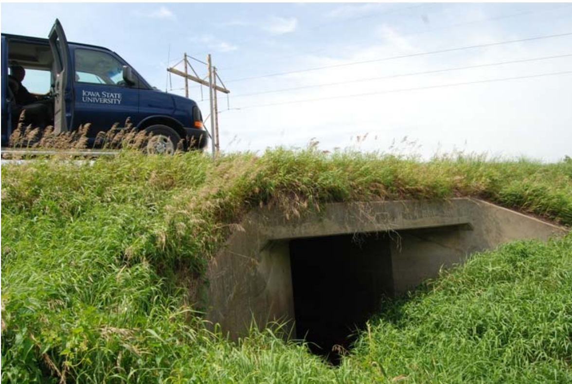
Figure A.6. Large culvert under IA 25
