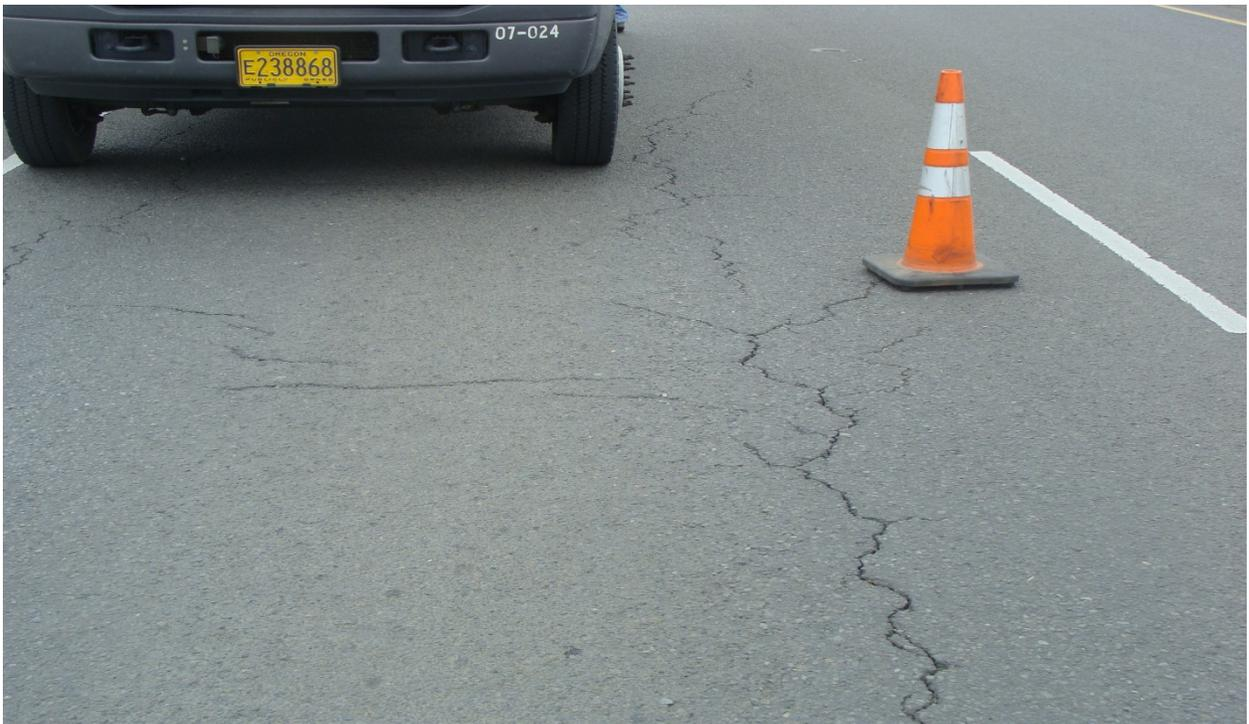
Figure 4.1: Top-Down and Transverse Cracking on Section OR238-C
