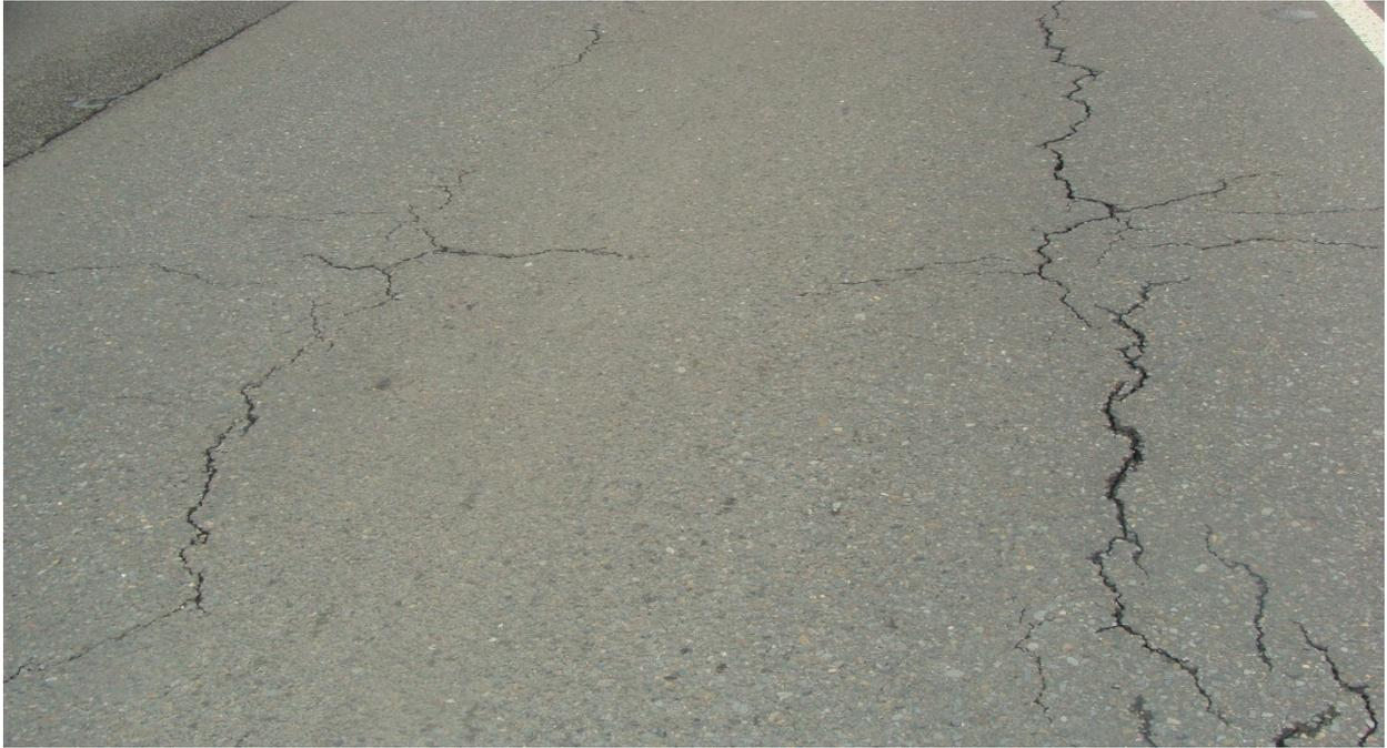
Figure 4.4: Top-Down and Transverse Cracking on Section OR99EB-C
