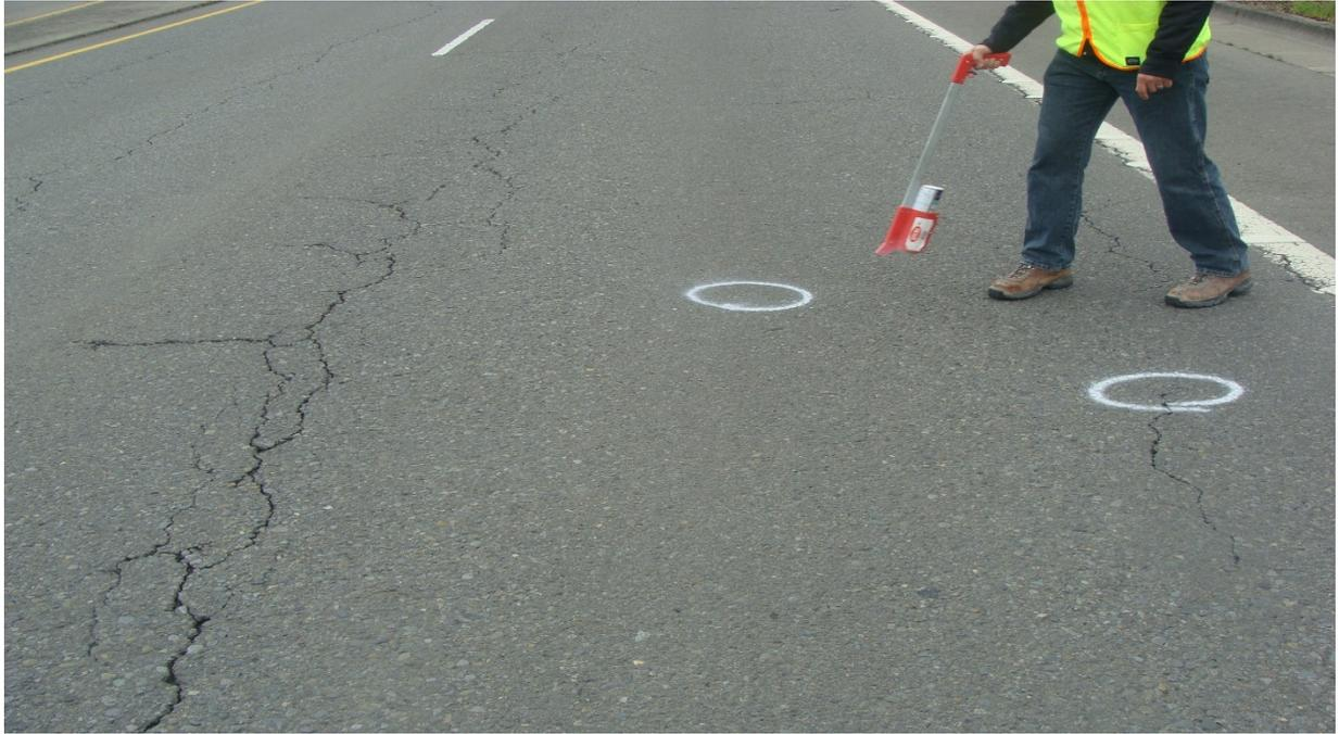
Figure 4.2: Top-Down Cracking on Section OR221-C
