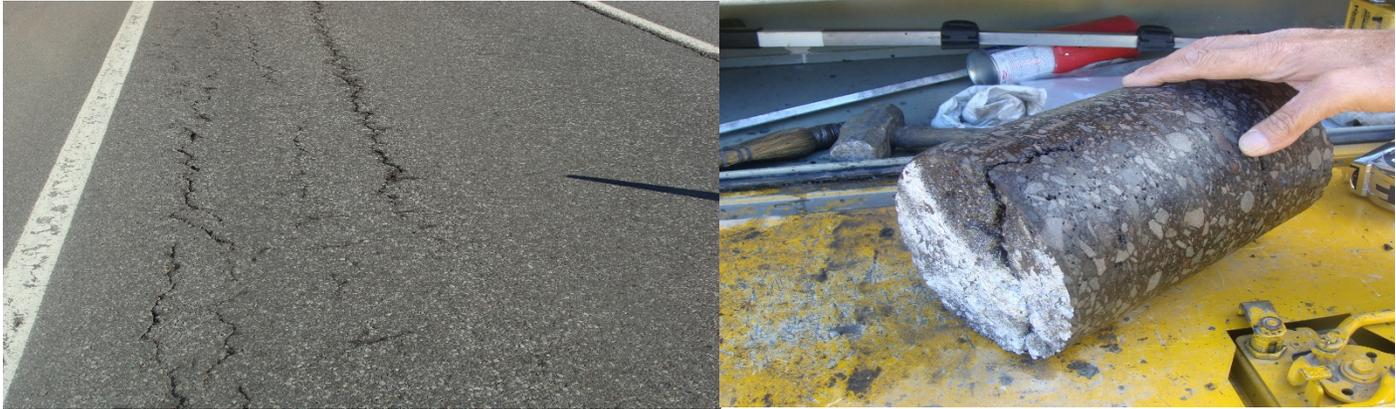
Figure 1.1: Pictures Showing the Development of Top-Down Cracking
