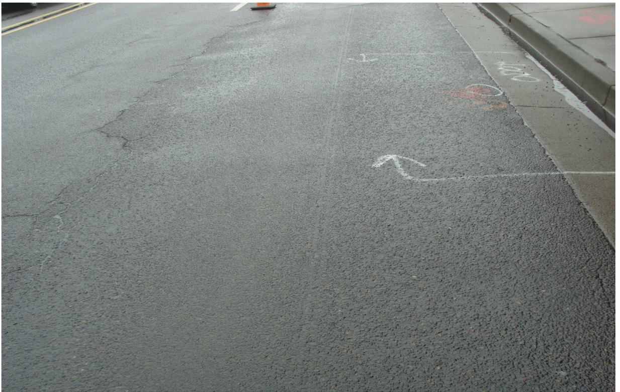
Figure 4.3: Tow-Down Cracking on Section OR99\*-C
