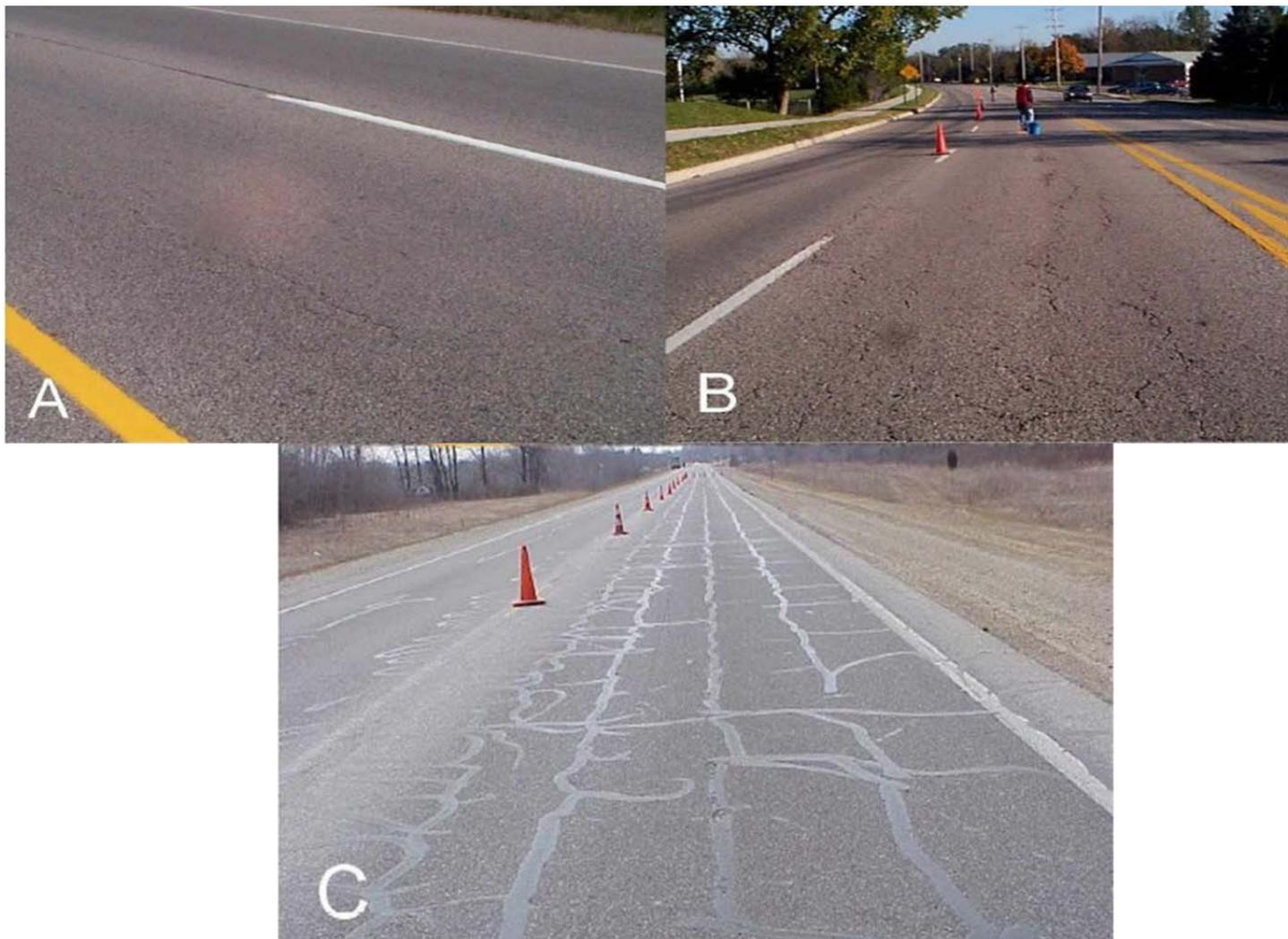
Figure 2.3: Photographs Illustrating the Development of Top-Down Cracking (Svasdisant *et al.*, 2002)
