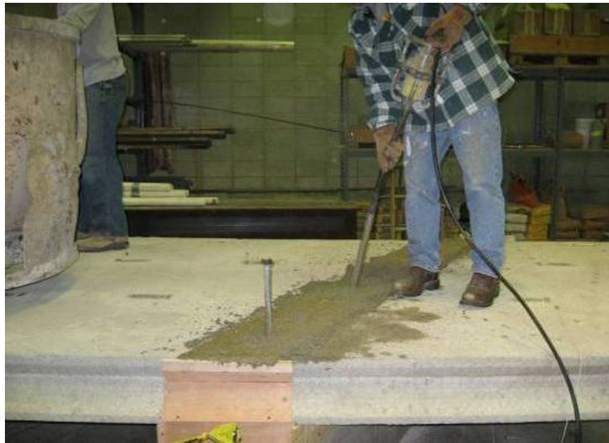
b) Placement of concrete in channel
