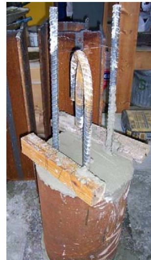
b) Pipe pile after placing concrete
