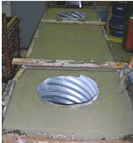
Figure 33. Abutment 6 after hand-finishing
