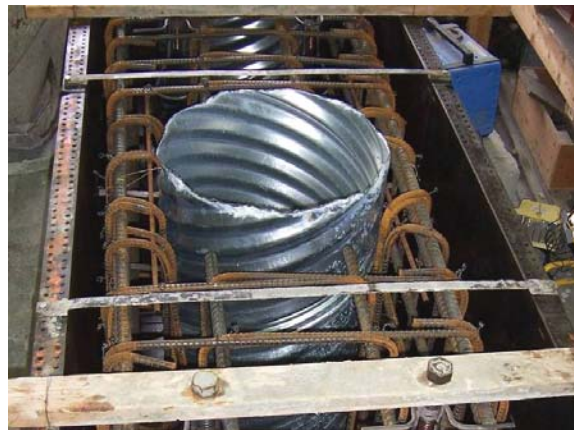
Figure 27. Pier cap reinforcement
