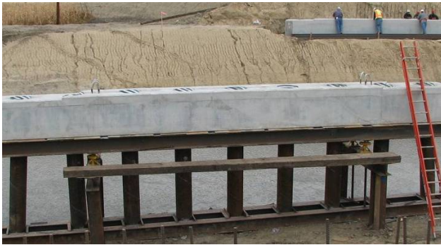
a) pier cap in place
