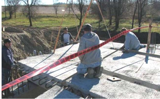
Figure 132. End panel being placed at the east end of the bridge, November 8
