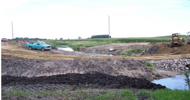
Figure 103. Cleared bridge site, August 7
