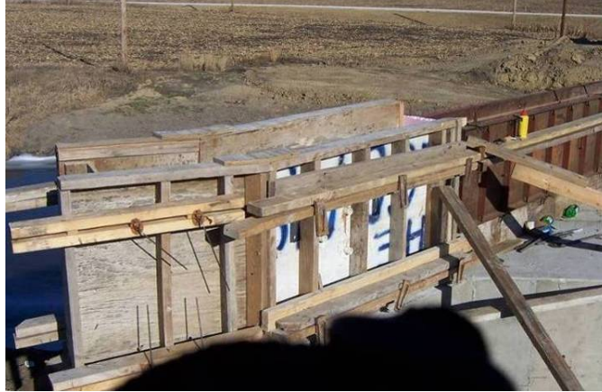
Figure 143. Barrier rail formwork, December 8
