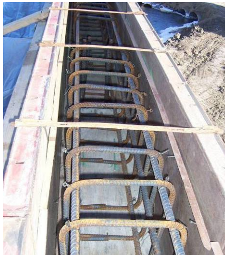
Figure 144. Barrier rail reinforcement, December 8
