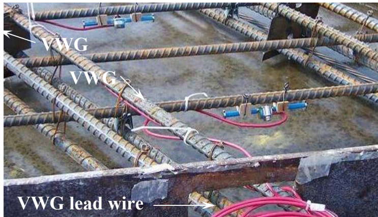
Figure 81. Deck panel vibrating wire gages
