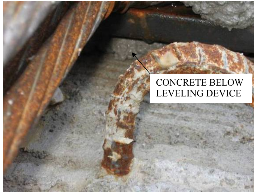
c) Concrete below the leveling device
