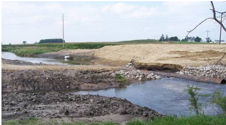
Figure 104. Access road and bridge site, August 11
