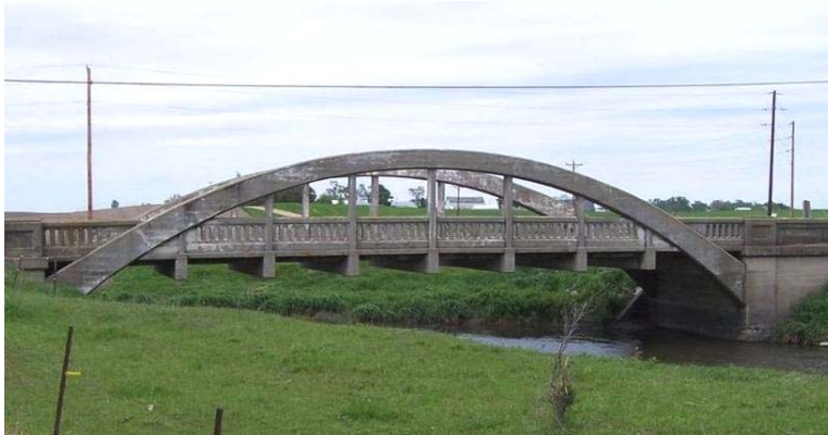
Figure 100. Previous bridge on 120 th Street, July 19
