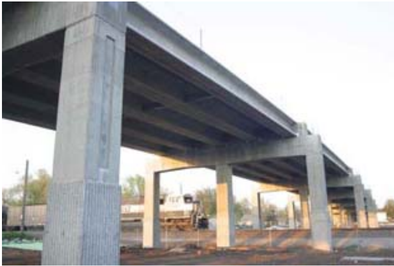
Figure 8. Bridge pier cap located Lincoln, Nebraska
