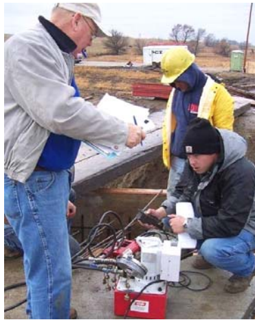
Figure 138. Post-tensioning in progress, November 28
