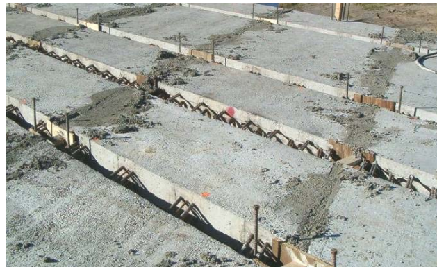
Figure 133. Several transverse joints before finishing, November 8
