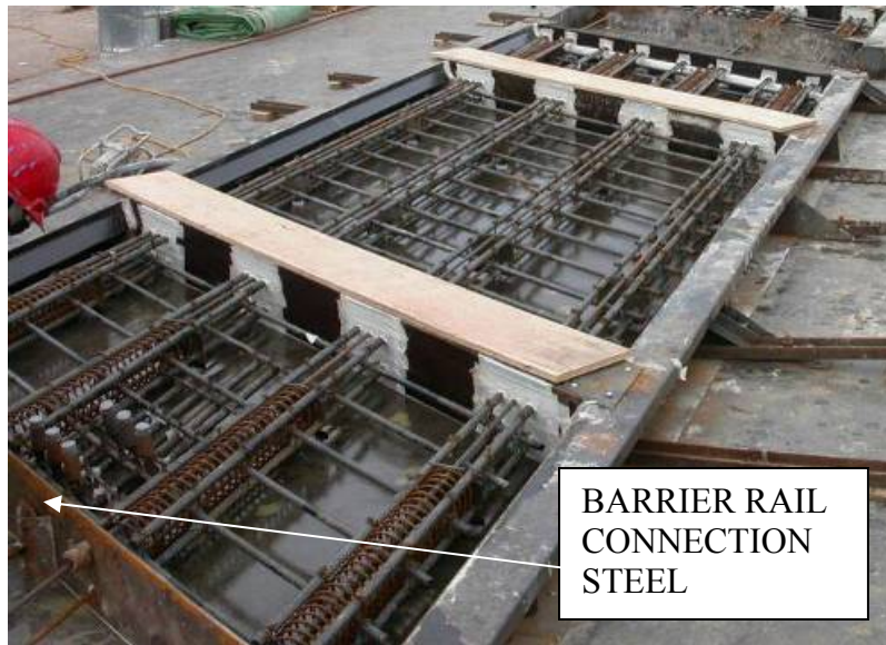
a) Deck panel reinforcing steel
