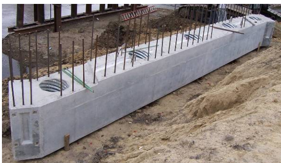
a) abutment in final position
