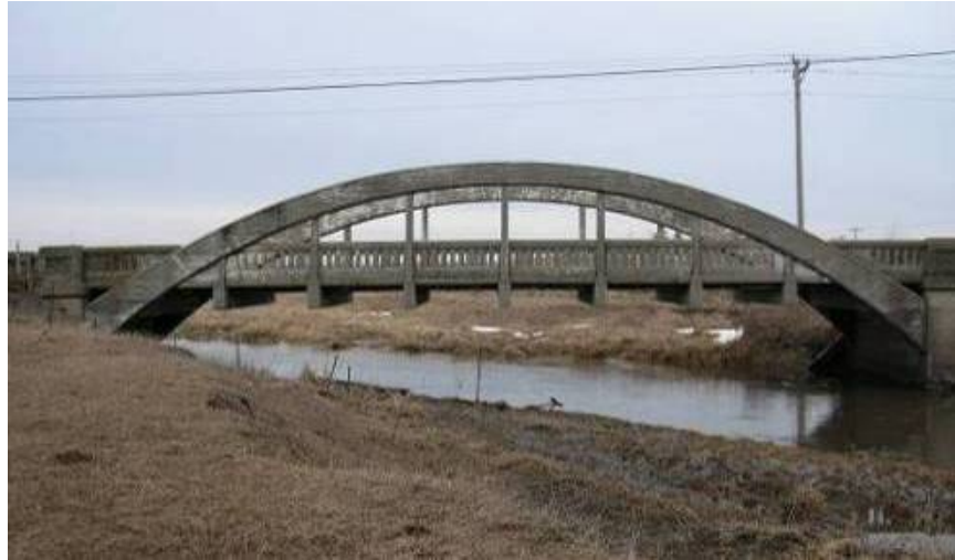
a) Replaced Marsh Arch bridge
