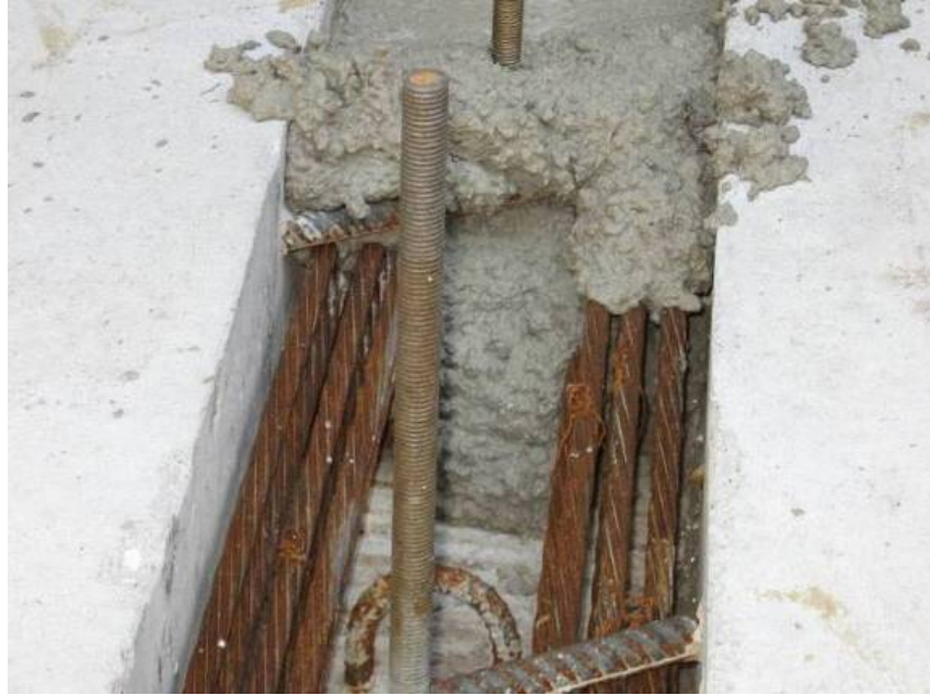
a) Concrete flowing in channel
