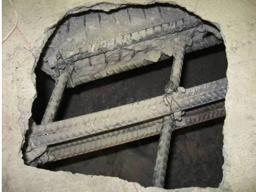
b) Top view after concrete removal
