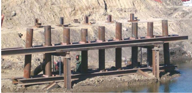
Figure 112. West pier and west abutment piling, September 28
