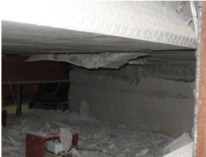
c) Underside of the deck panel
