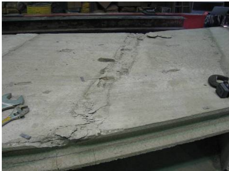
a) Deck panel after loading
