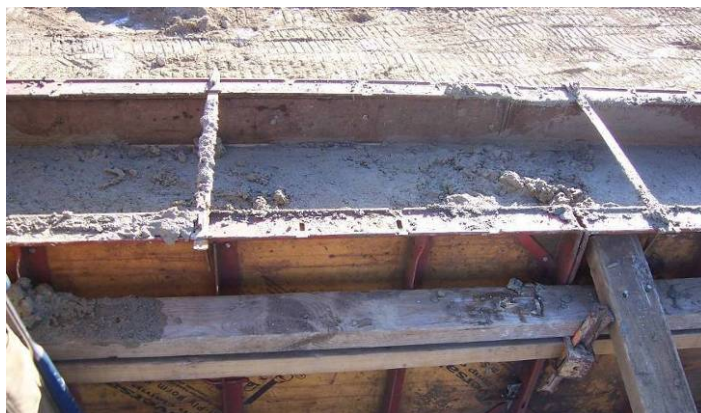
Figure 145. Barrier rail before final finishing, December 8
