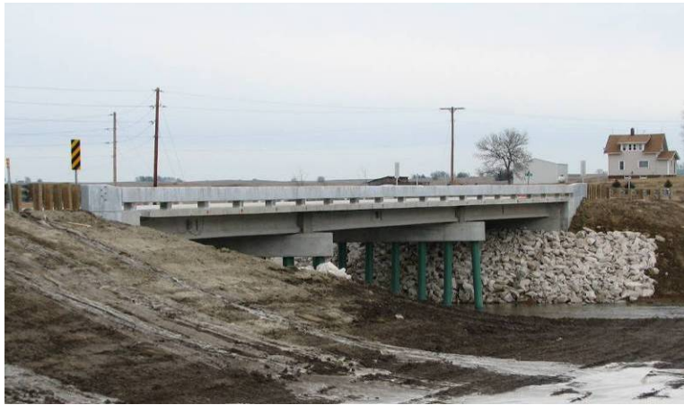
Figure 149. Completed bridge, December 27
