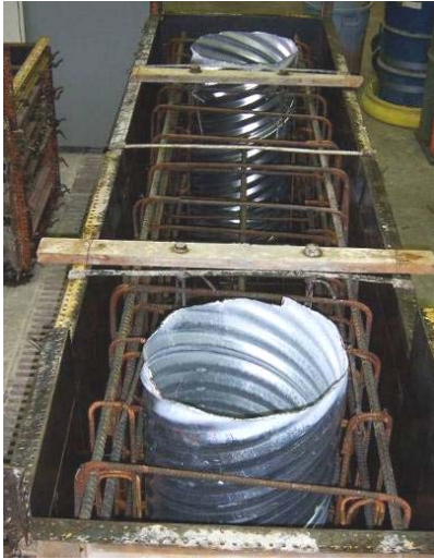
Figure 32. Finished reinforcement and formwork for ADC1
