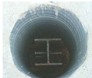
b) H-pile in the abutment
