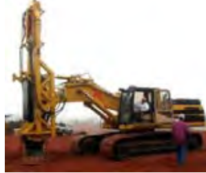
Figure 1. The Rapid Impact Compactor (Courtesy of GeoStructures, Inc.)
