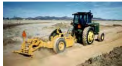
Figure 3. Impactor 2000 "square" impact roller (Courtesy of Impact Roller Technology, Nebraska)
