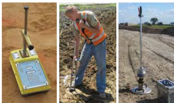
Figure 2. Nuclear gage (top left), dynamic cone penetrometer (top right), light weight deflectometer (bottom)
