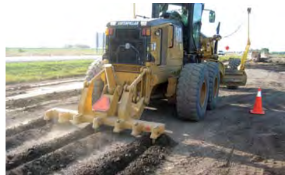
Figure 3. Preparation of calibration test beds
