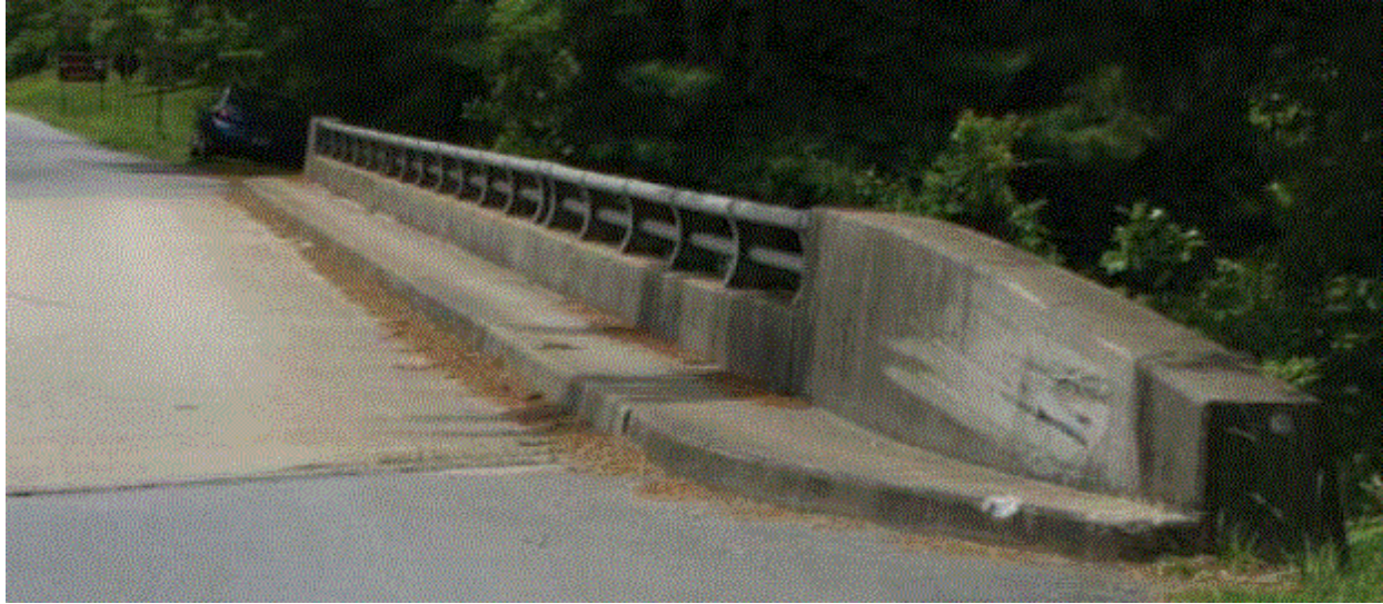
Figure 1. Unshielded bridge rail end
