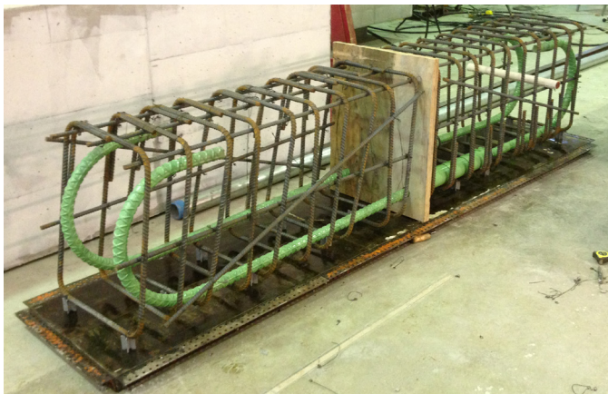
Formwork, reinforcing cage, and #14 bars and couplers for laboratory specimens during construction
