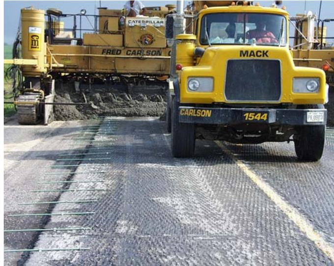
**Figure 10. Stapped #4 Bar that Ties the Widening Unit to the Thin Overlay**
