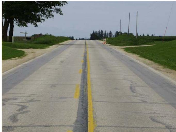
**Figure 3. Longitudinal Cracking and Current Condition of the Roadway**
