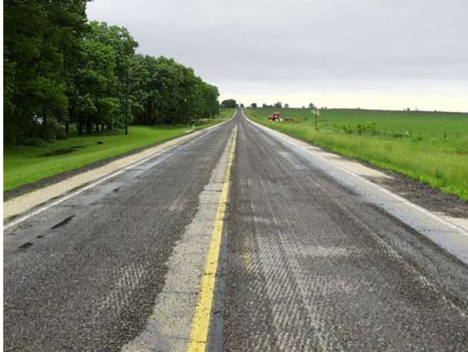
**Figure 5. Scarified Pavement Surface**
