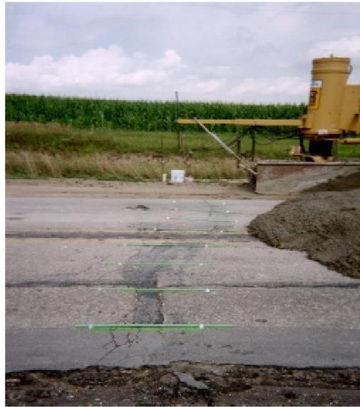
**Figure 8. Tied Transverse Crack**
