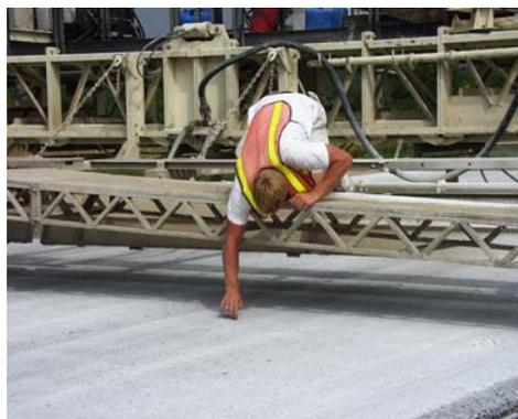
**Figure A.2. Iowa Maturity Device Installation**
