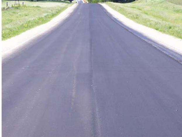
**Figure 7. HMA Stress Relief Layer**
