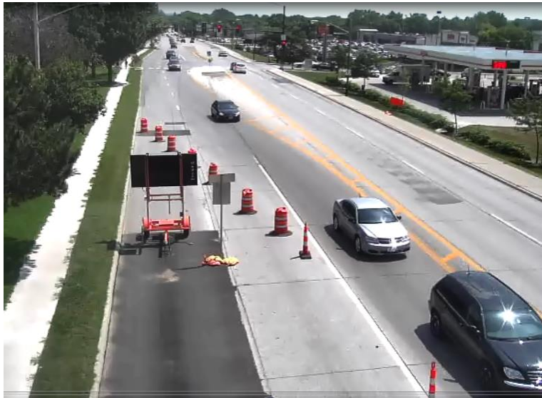
Figure 12. Camera view of drivers merging in work zone
