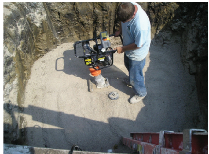
Compaction to achieve relative density higher than 35% (medium to dense material)
