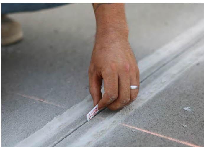
Figure 30. Using temporary joint spacers to protect and minimize damage due to early entry sawing (Source: Husqvarna)
