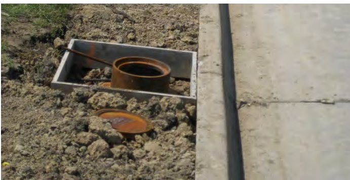
Figure 35. Subdrain retrofit operation including cleanout (The Transtec Group)
