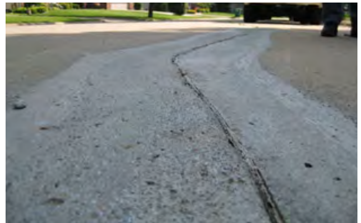
Figure 39. Completed patch (Source: The Transtec Group)
