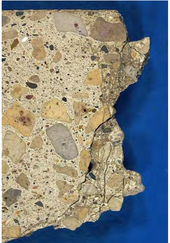
Figure 23. Deterioration due to bottom-up moisture
