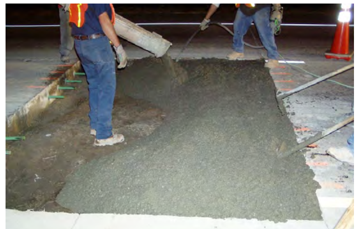
Figure 40. Full-depth patching
