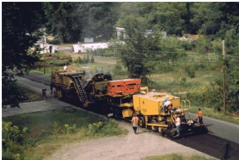
Figure 9. Cold in-place recycling
