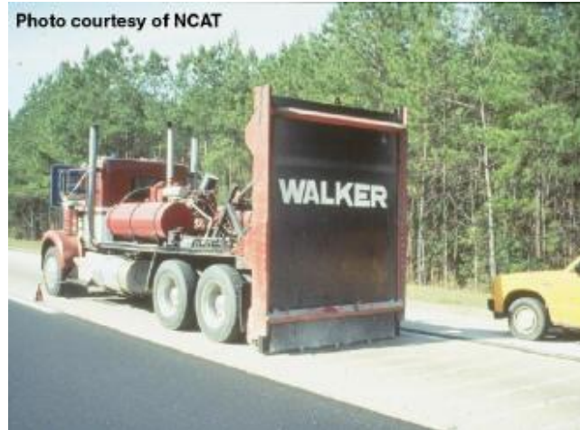
Figure 3. Crack and seat
