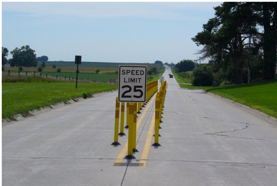
Figure 21: Creation of a center island with channelizers
