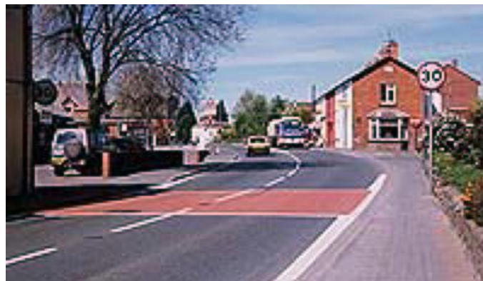
Figure 45: Treatment used in Shropshire, UK (DETR, 2005)
