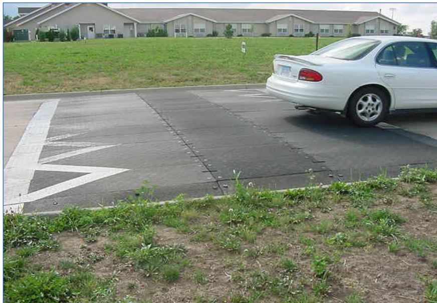
Figure 13: 30 mph speed table in study for residential traffic calming in small Iowa communities
