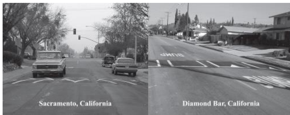
Figure 14: Typical asphalt speed lumps in California (Gulden and Ewing, 2009)
