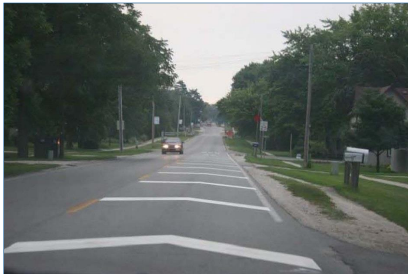
Figure 39: Use of converging chevrons on County Road E-18 in Iowa
