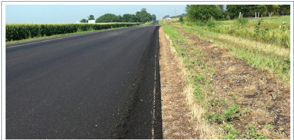
Figure 1. HMA Safety Edge in Kossuth County, Iowa
