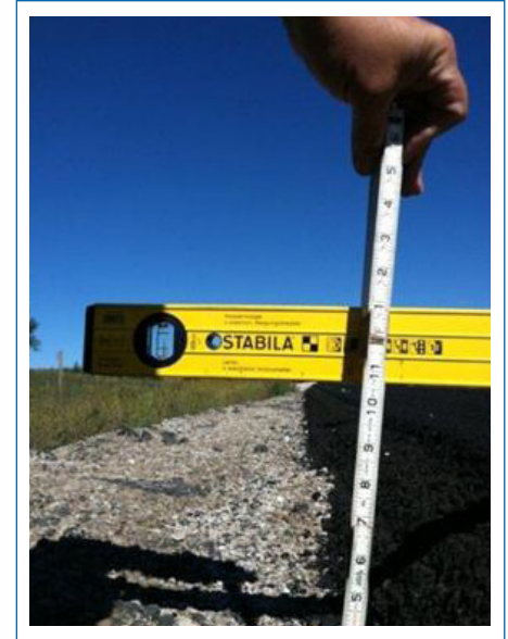
Figure 5. Severe pavement edge drop-off (10-12 inches)
