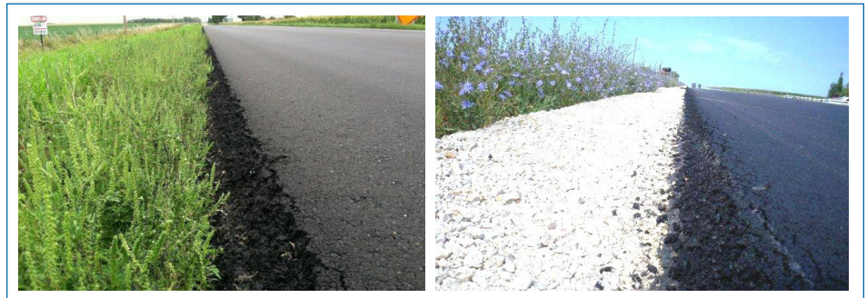
Figure 2. Insufficient base widths
