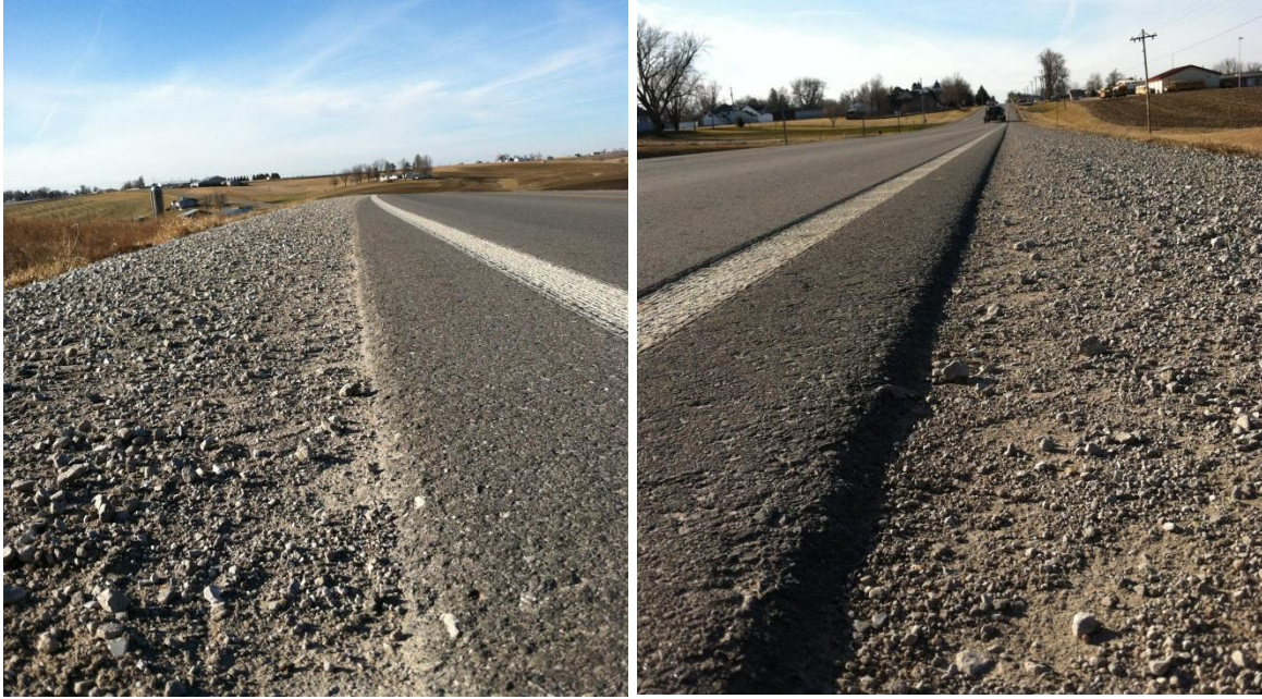
Figure 8. Typical shoulder degradation for HMA pavements with the Safety Edge (left) and with less than 30 degree slope (right)
