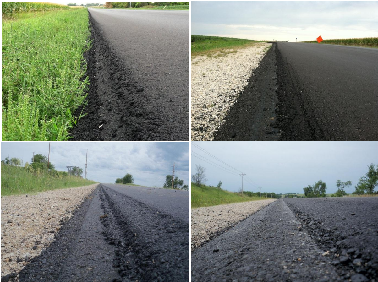
Figure 12. Excess base width examples
