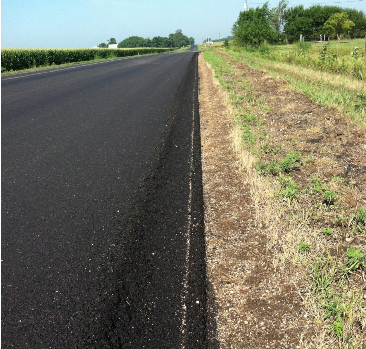
Figure 1. HMA Safety Edge in Kossuth County, Iowa
