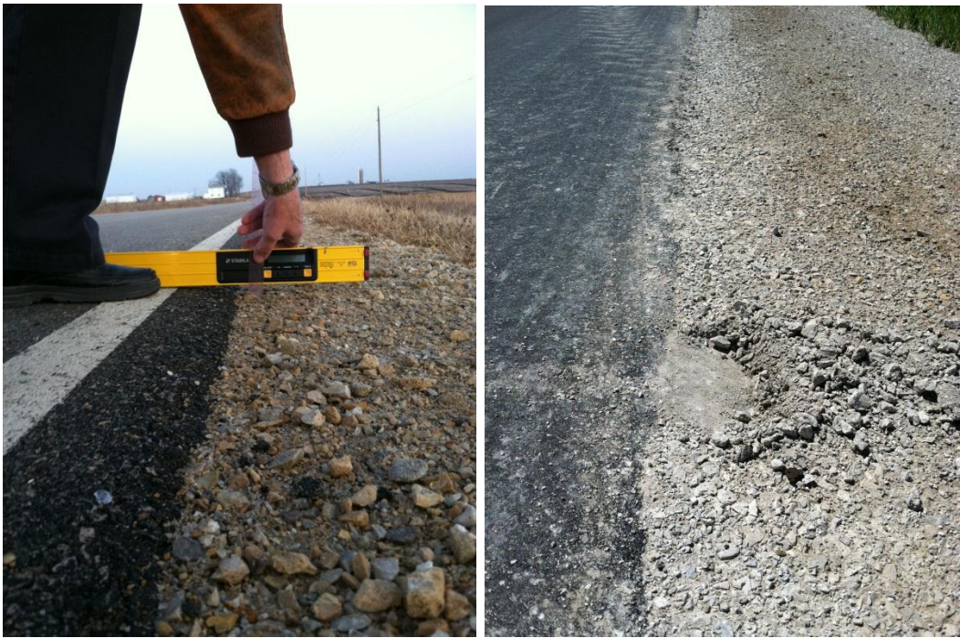
Figure 10. Exposed Safety Edge slope faces
