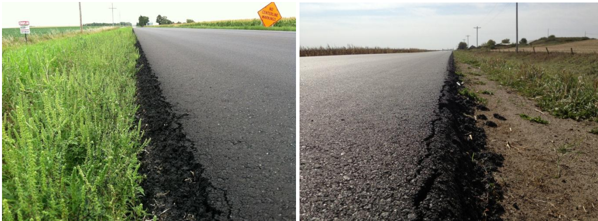
Figure 13. Insufficient base width examples
