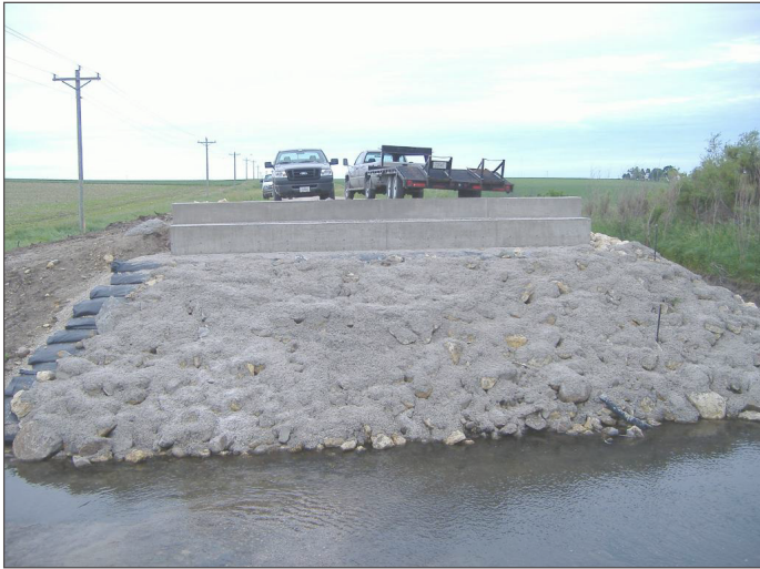
Figure 1. Bridge 1 GRS abutment with grouted riprap facing
