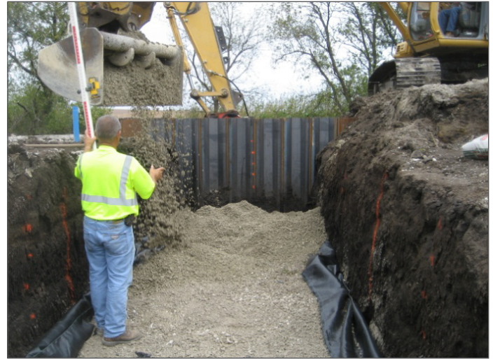
Figure 2. Bridge 2 GRS fill material placed to support footing
