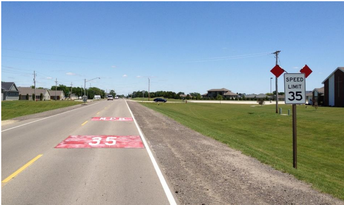
Figure 5-5: Colored entrance treatment for Jesup west entrance
