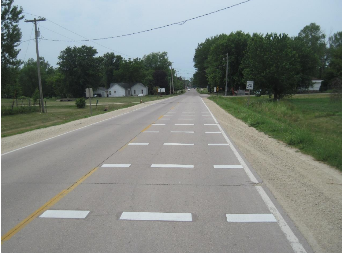
Figure 5-2: Transverse bar treatment at Hazleton east entrance
