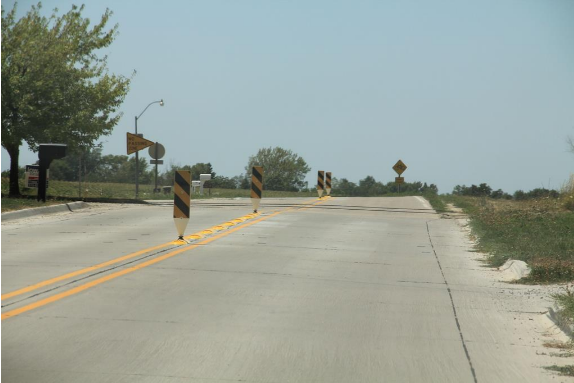
Figure 5-15: Mountable curbing installed at west St. Charles community entrance
