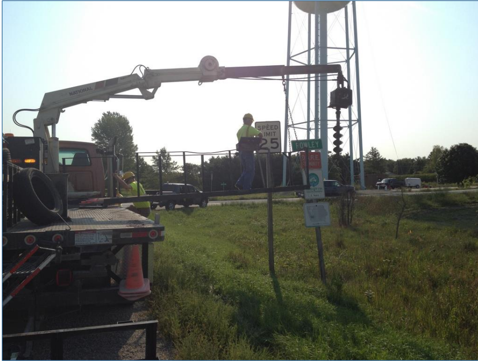
Figure 3-13: Installation of LED speed limit sign
