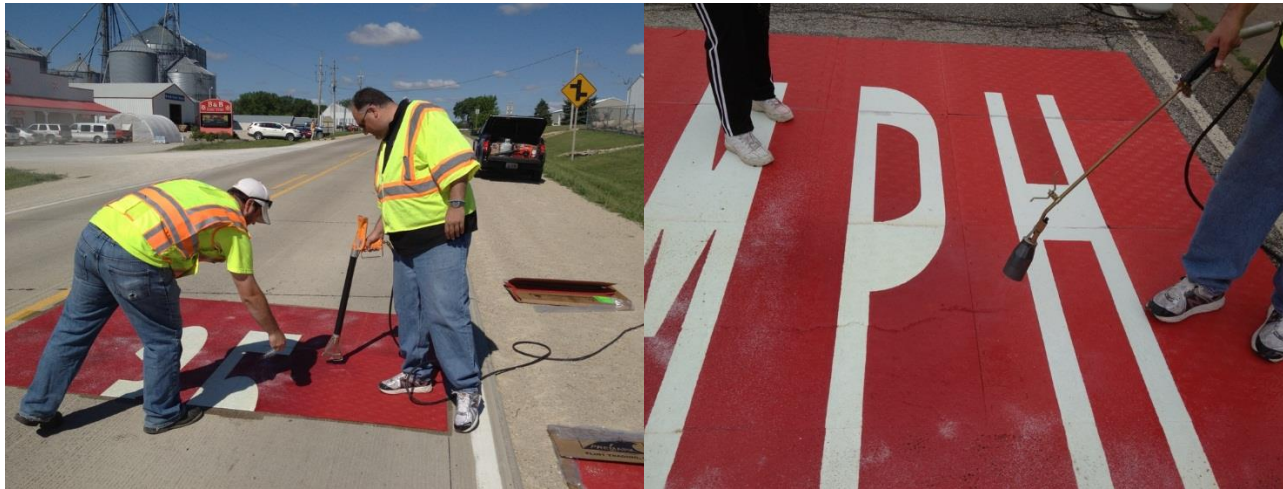
Figure 3-8: Installation of colored entrance treatment
