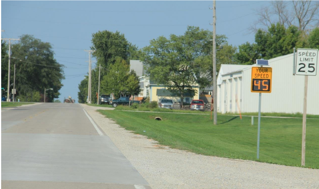
Figure 5-19: DSFS installed at east Rowley community entrance
