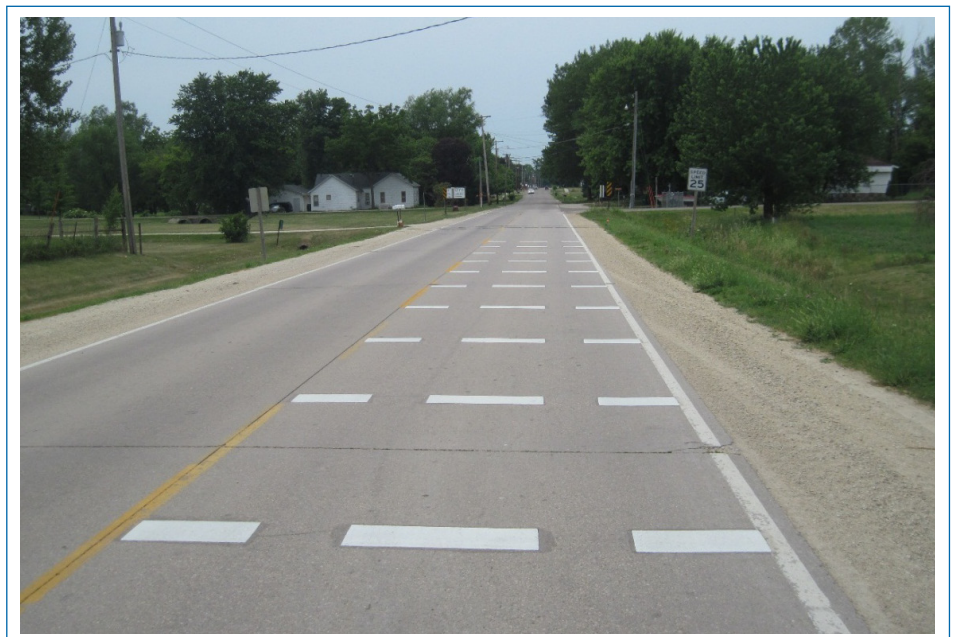
Transverse bar treatment at Hazleton east entrance
