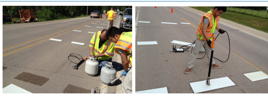
Application of transverse bar treatments
