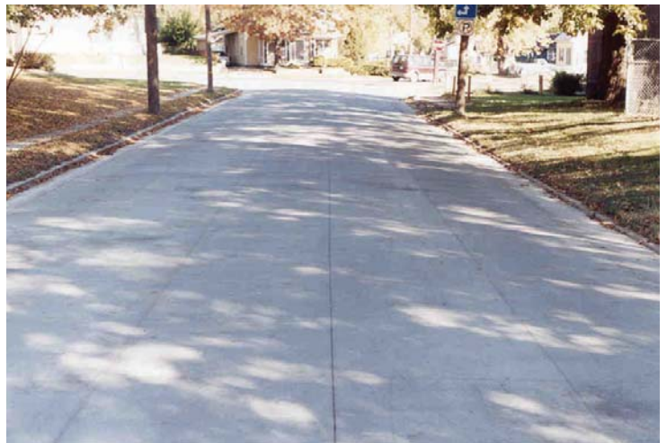
Completed overlay paving for the Des Moines project
