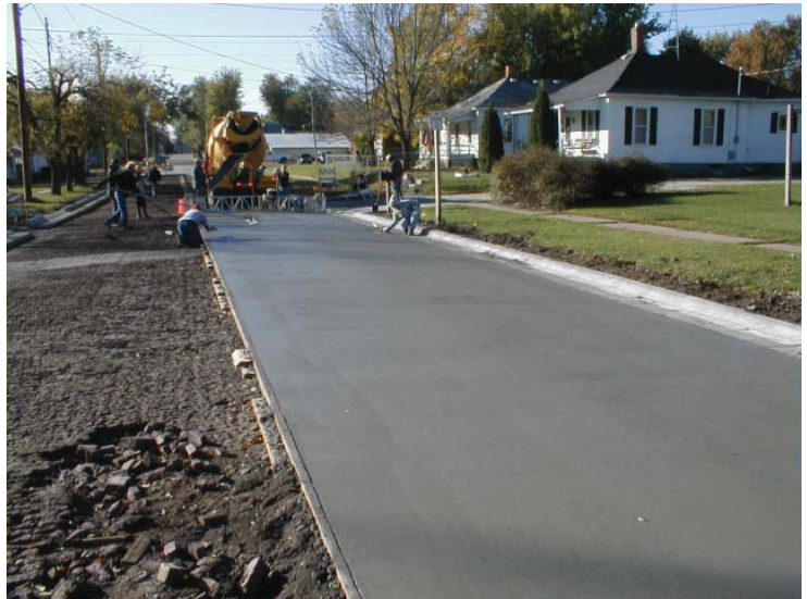
Overlay paving on the Oskaloosa project
