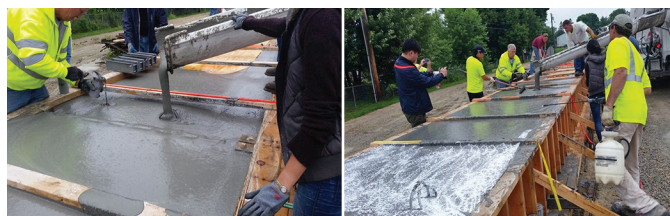
Pouring the K-UHPC mix into the formwork
