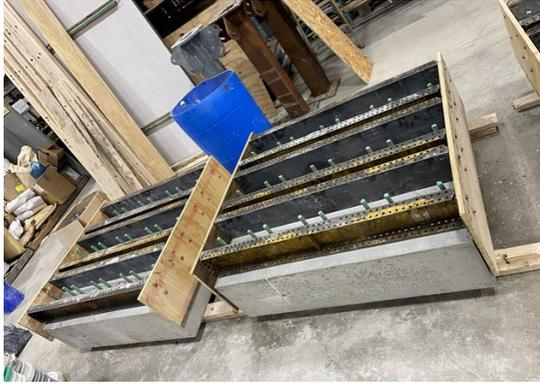
**Building the formwork to cast the filling**
