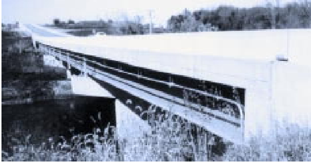
FIGURE 1 Boone River bridge on IA-17.
