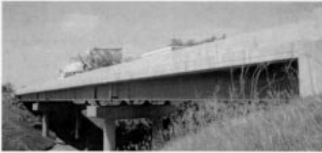
FIGURE 2 I-80 Bridge No. 7804.8L080.
