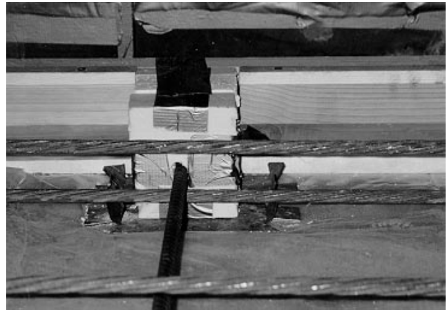
FIGURE 7 Shear-key and pocket forming.
