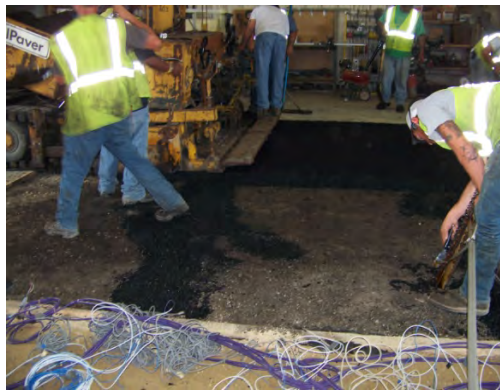
Figure 3. Paving test sections
