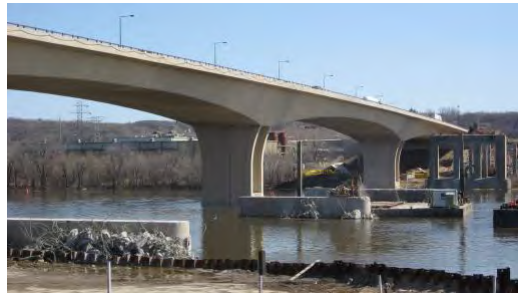
Figure 1: Westbound lanes of the Wakota Bridge completed, the eastbound lanes were completed and opened in 2010
