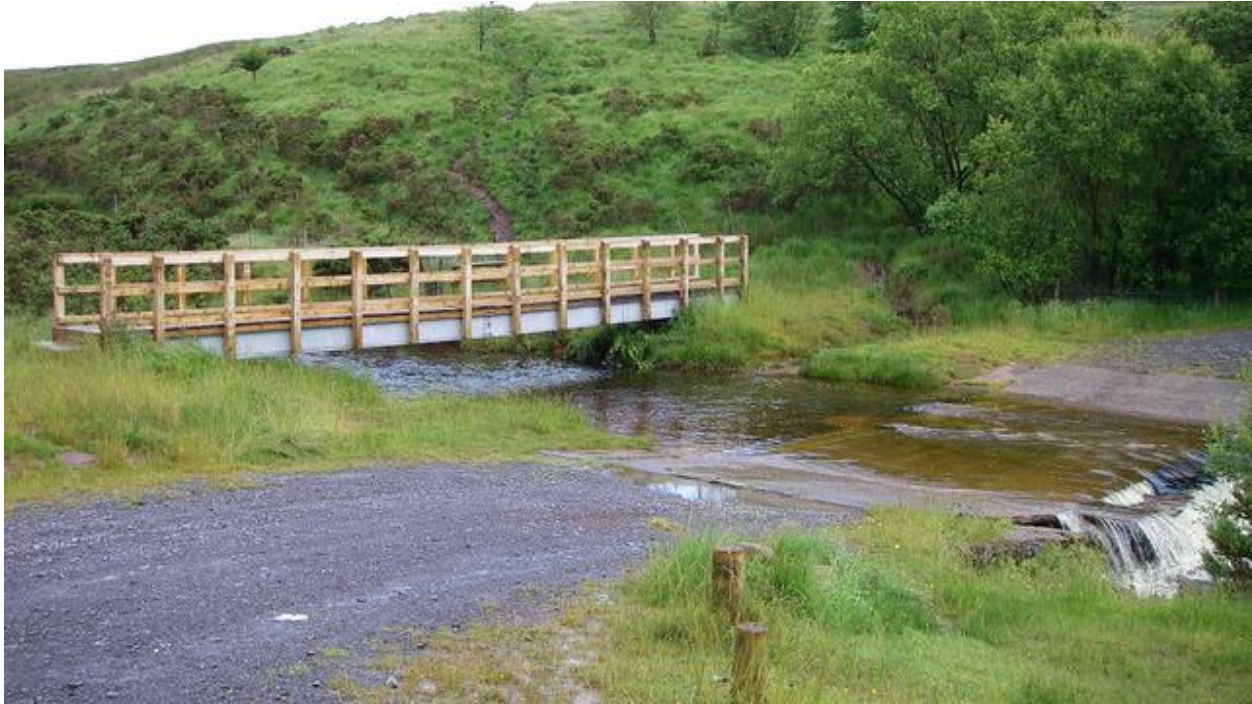
Figure 5. Low-water crossings and pedestrian bridges can be an inexpensive way to provide secondary access to an area that has the potential to be cut off by an adverse event.
